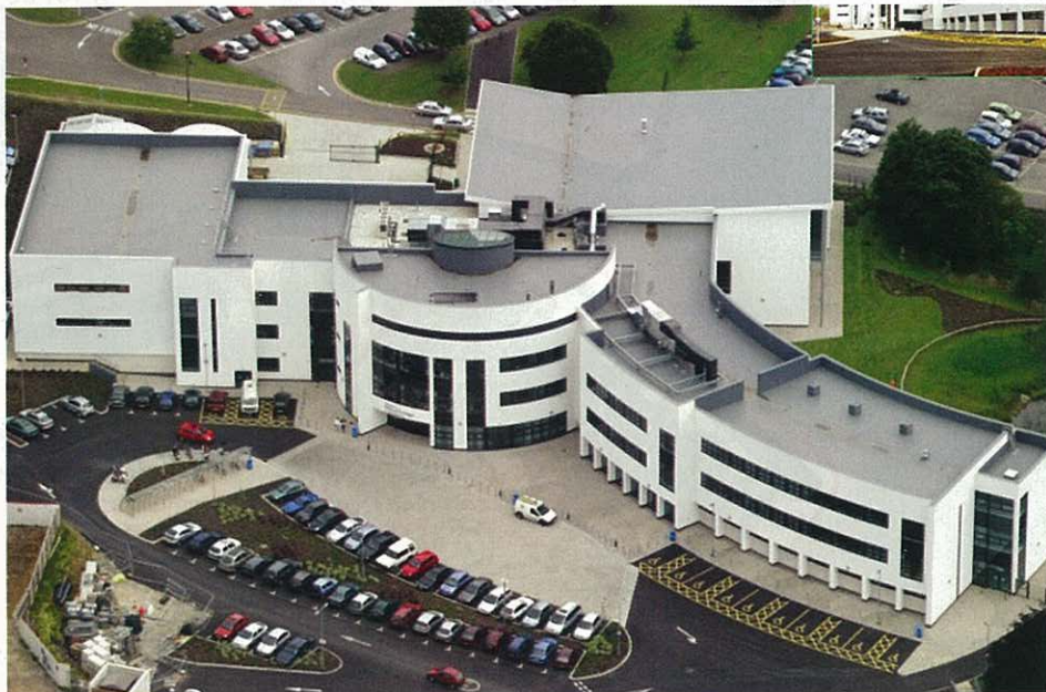
The roof at Stroud College demonstrates the impressive finish that single ply can deliver.
