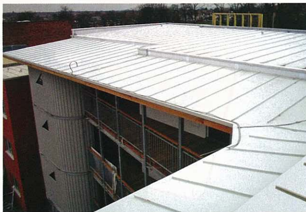
Wood Green Apartments: an example of single ply being used to replicate standing seam.
